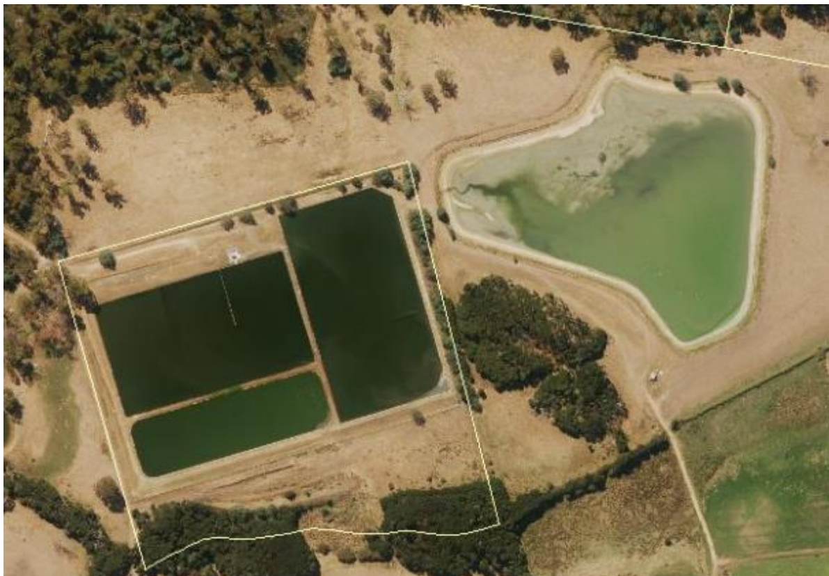
Figure 30.-1: Legana Sewage Treatment Plant
