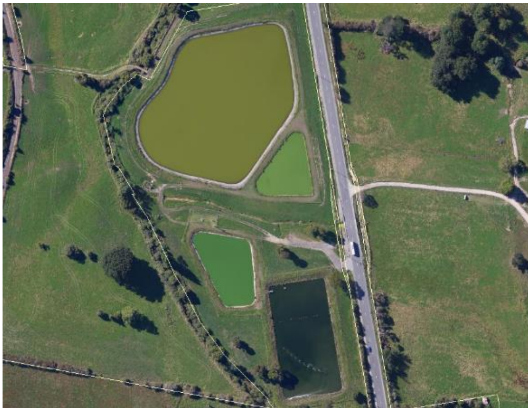
Figure 31-1: Lilydale Sewage Treatment Plant
