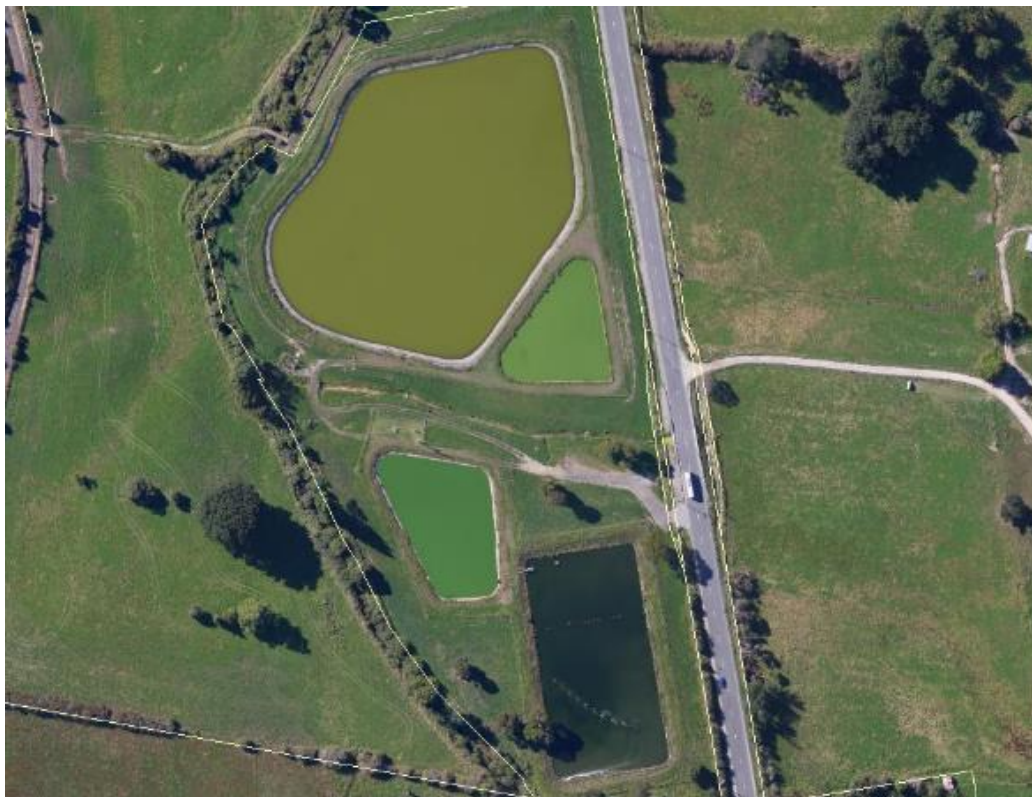
Figure 31-1: Lilydale Sewage Treatment Plant
