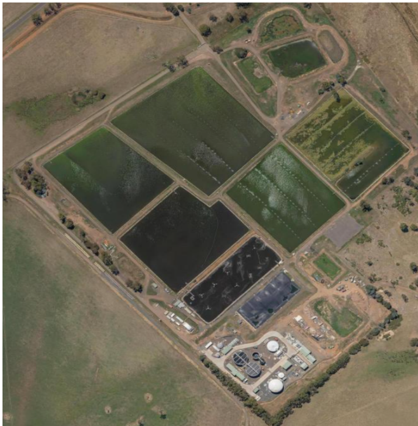
Figure 32-1: Longford Sewage Treatment Plant
