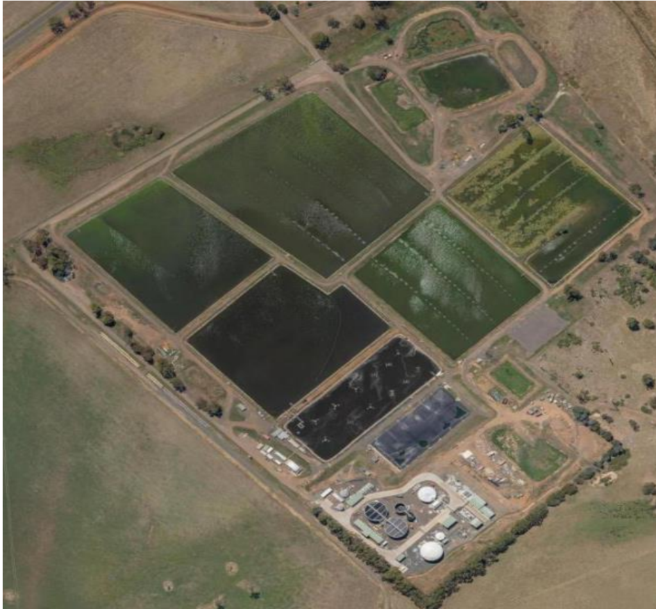
Figure 32-1: Longford Sewage Treatment Plant
