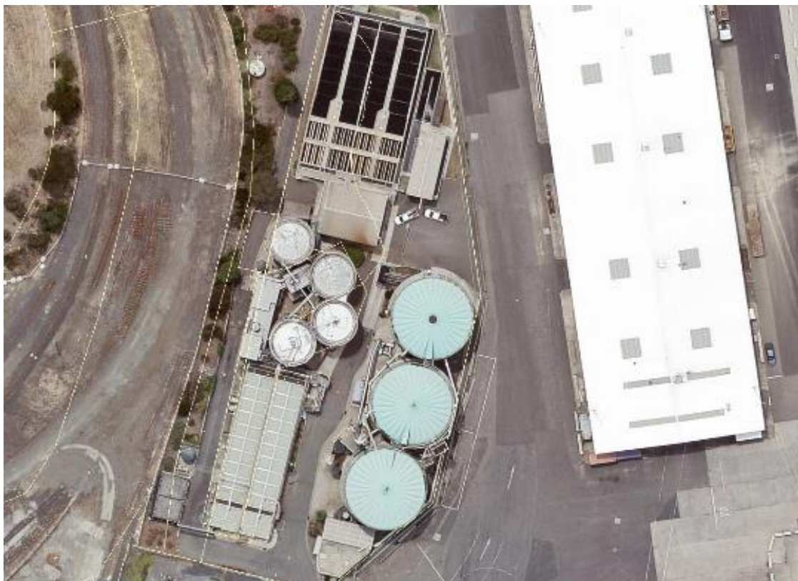
Figure 33-1: Macquarie Point Sewage Treatment Plant
