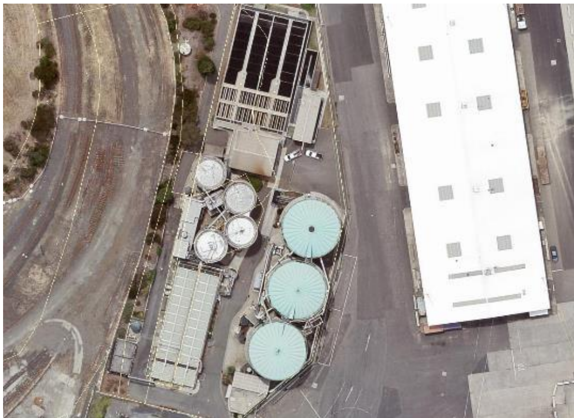
Figure 33-1: Macquarie Point Sewage Treatment Plant
