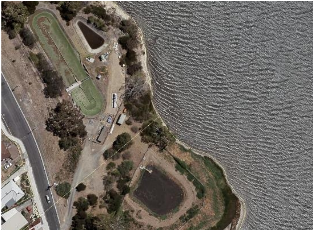
Figure 34–1: Midway Point Sewage Treatment Plant
