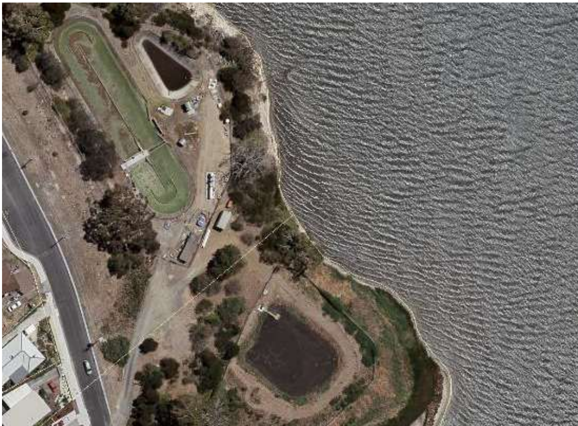
Figure 34-1: Midway Point Sewage Treatment Plant
