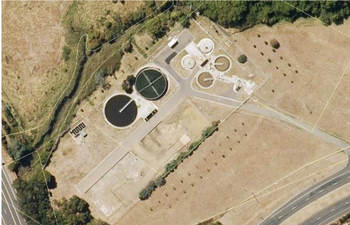
Figure 35-1: Newnham Sewage Treatment Plant
