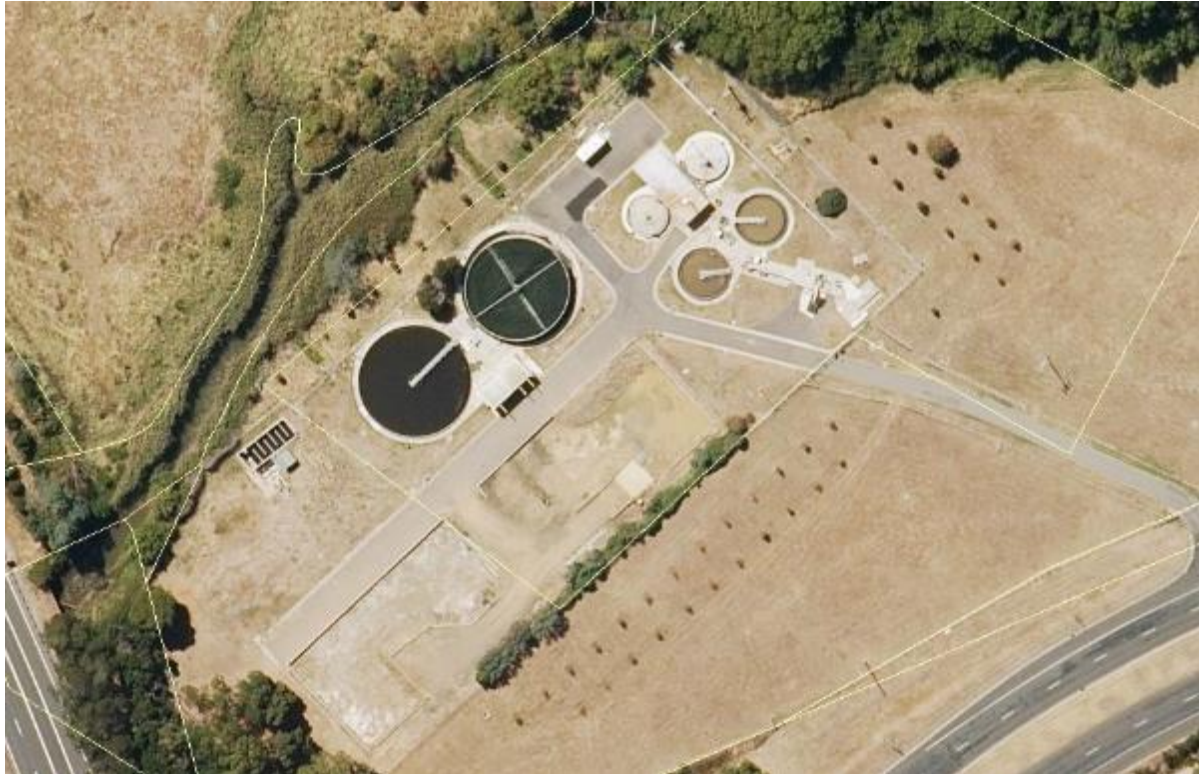
Figure 35-1: Newnham Sewage Treatment Plant
