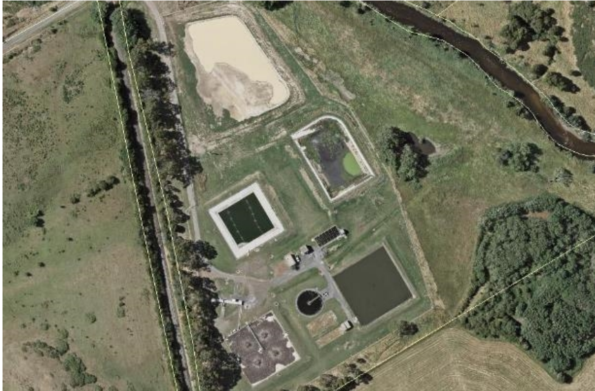
Figure 36-1: Norwood Sewage Treatment Plant
