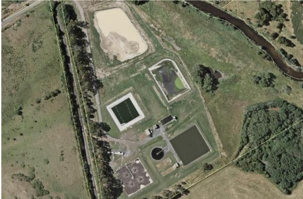
Figure 36-1: Norwood Sewage Treatment Plant
