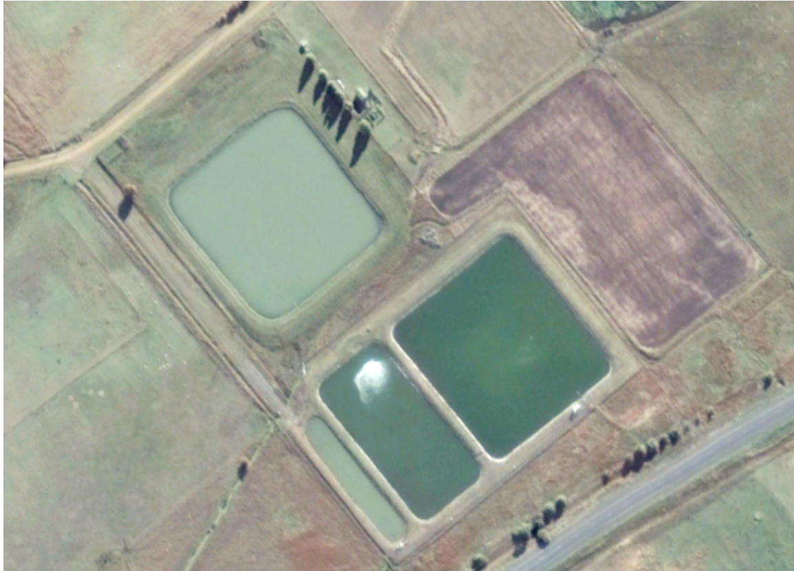
Figure 37-1: Oatlands Sewage Treatment Plant
