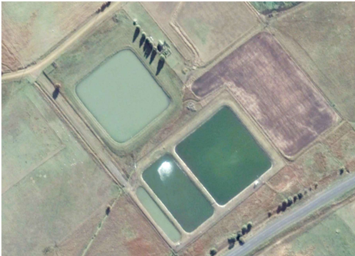
Figure 37-1: Oatlands Sewage Treatment Plant
