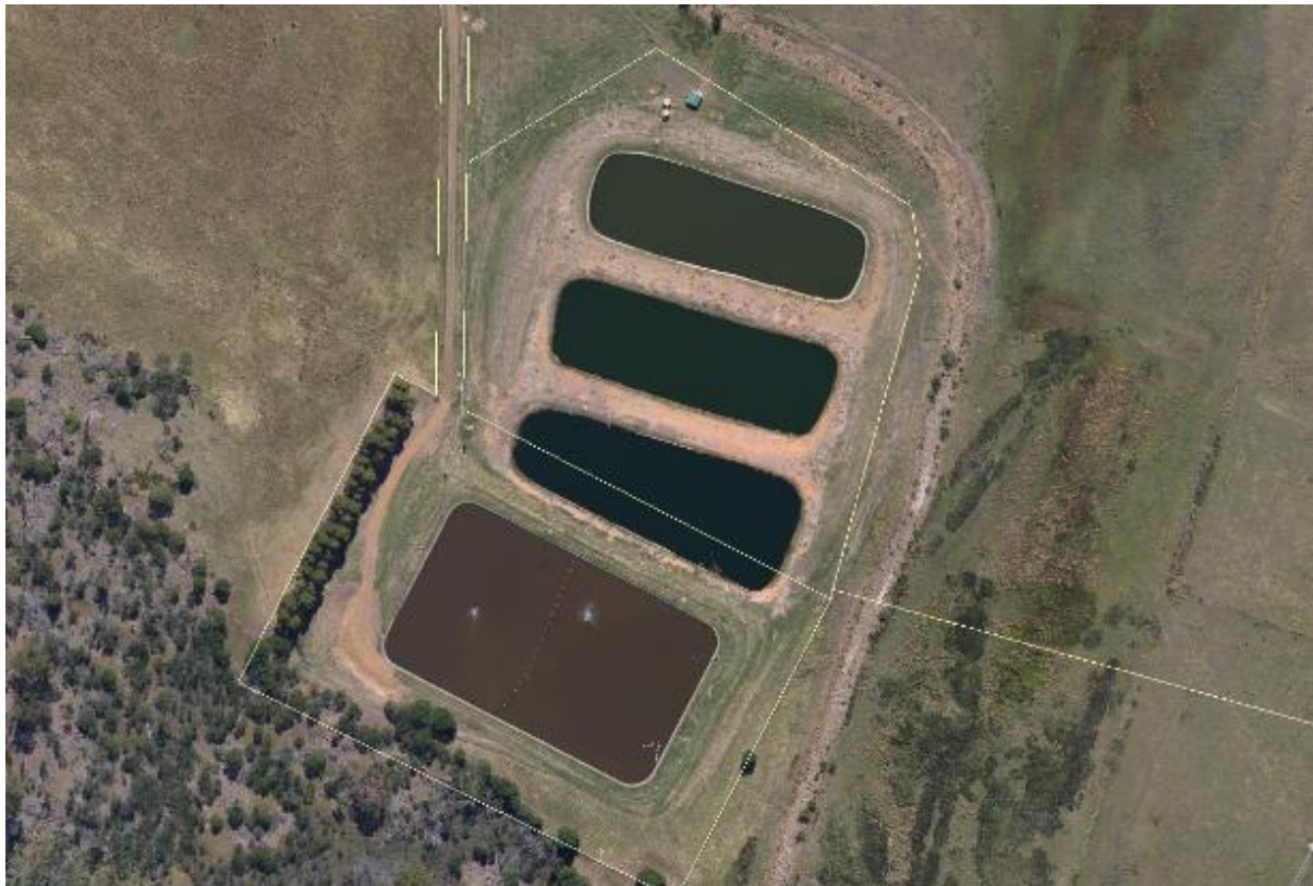
Figure 38–1: Orford Sewage Treatment Plant
