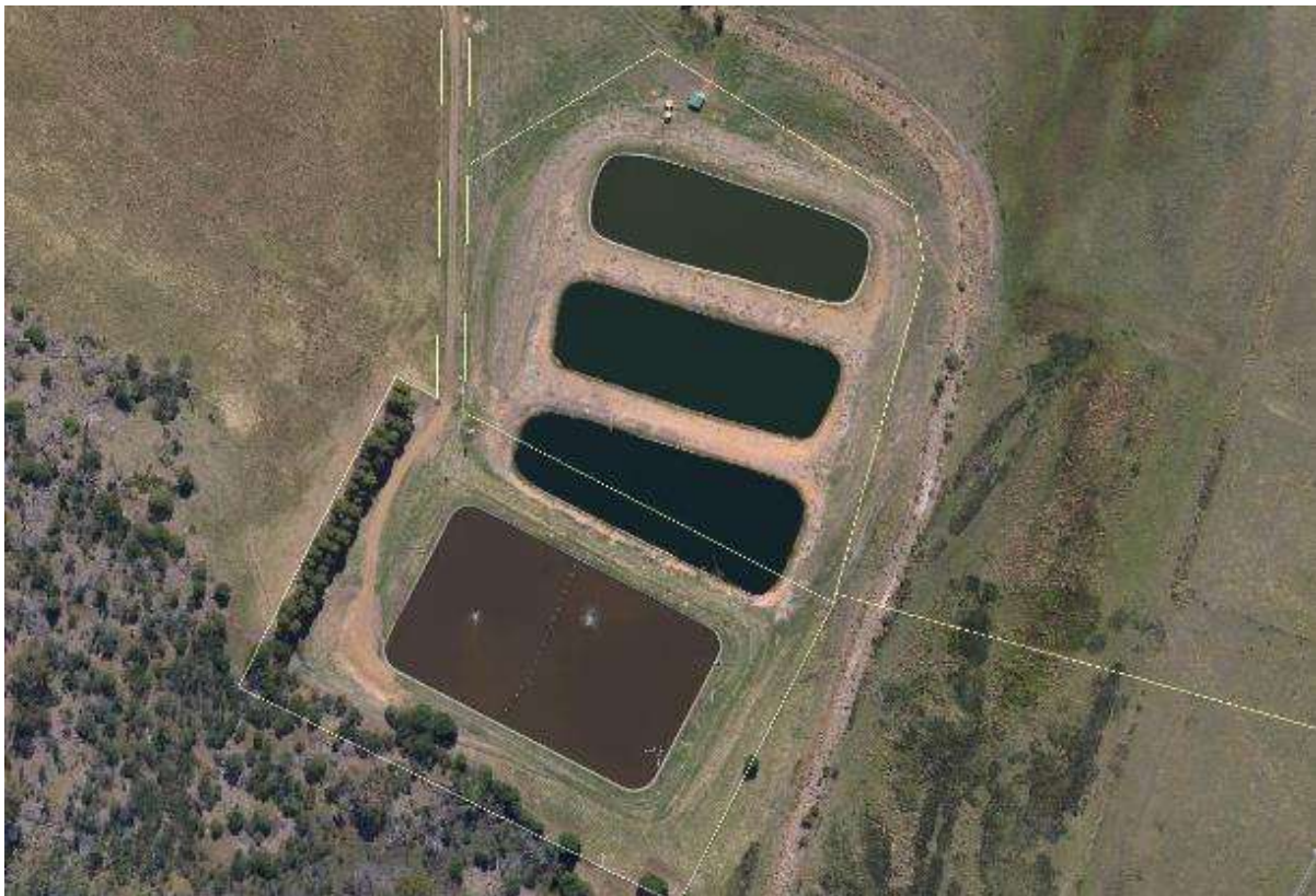
Figure 38-1: Orford Sewage Treatment Plant
