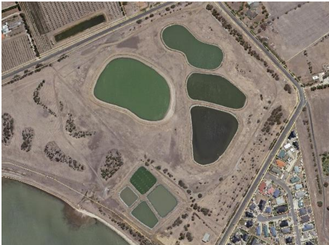
Figure 40-1: Penna Sewage Treatment Plant
