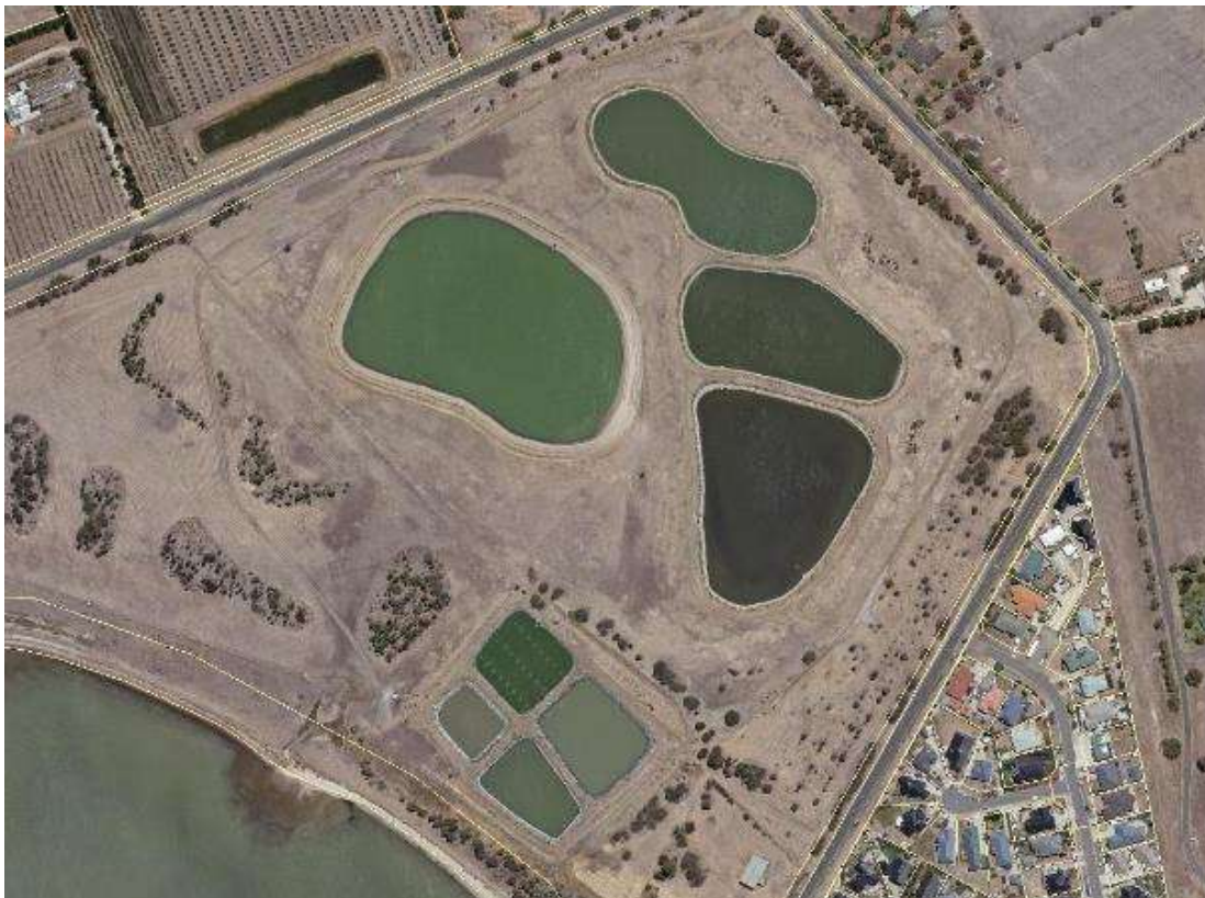
Figure 40-1: Penna Sewage Treatment Plant
