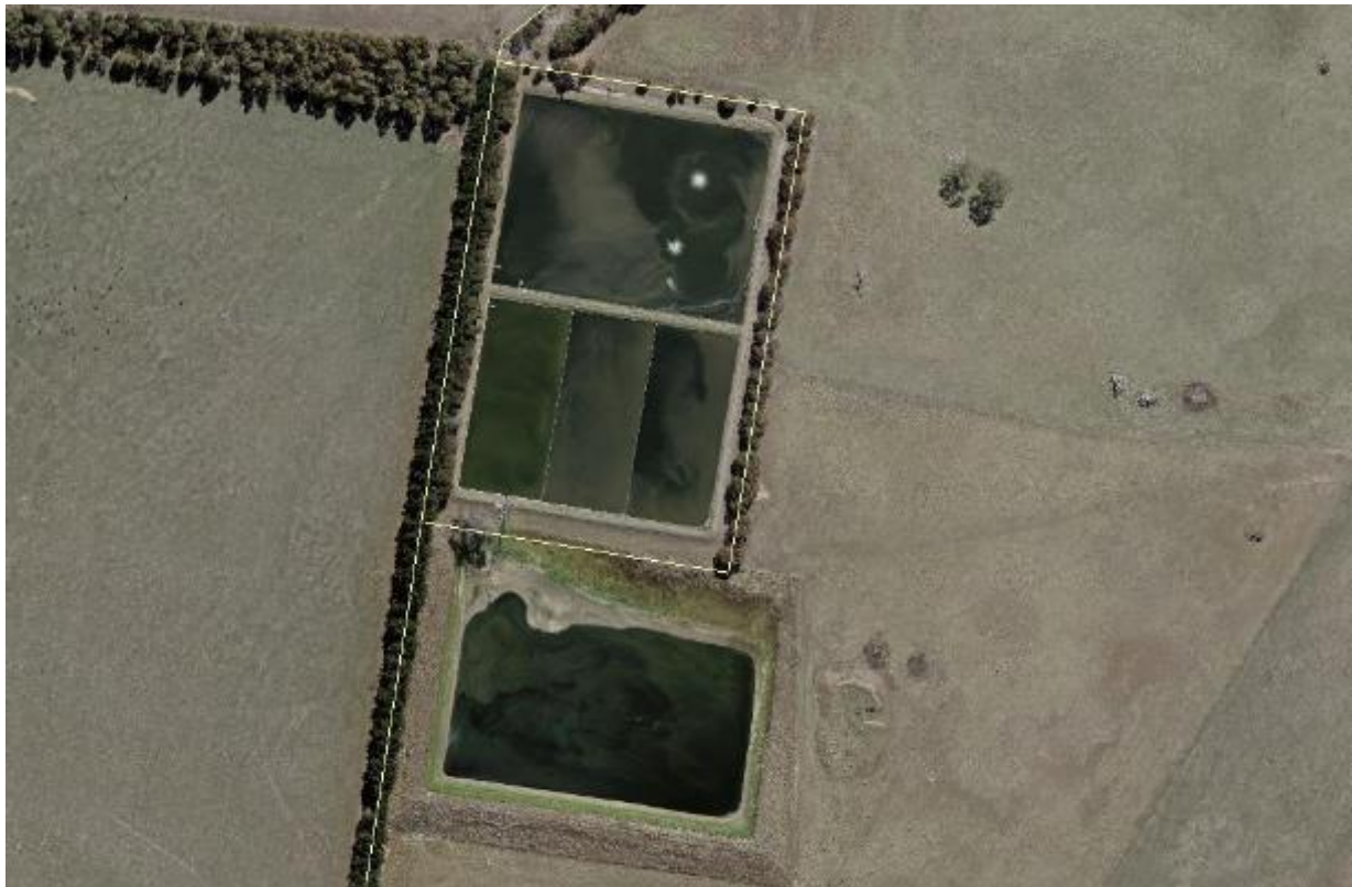
Figure O-1: Perth Sewage Treatment Plant
