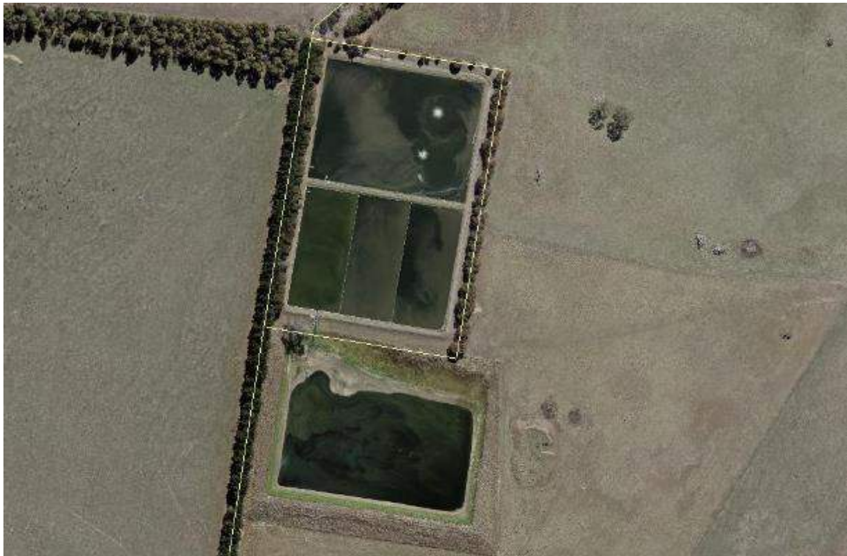
Figure O-1: Perth Sewage Treatment Plant
