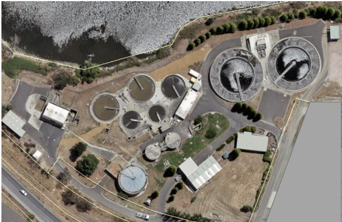
Figure 43- 1: Prince of Wales Sewage Treatment Plant
