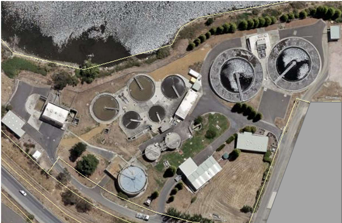
Figure 43- 1: Prince of Wales Sewage Treatment Plant
