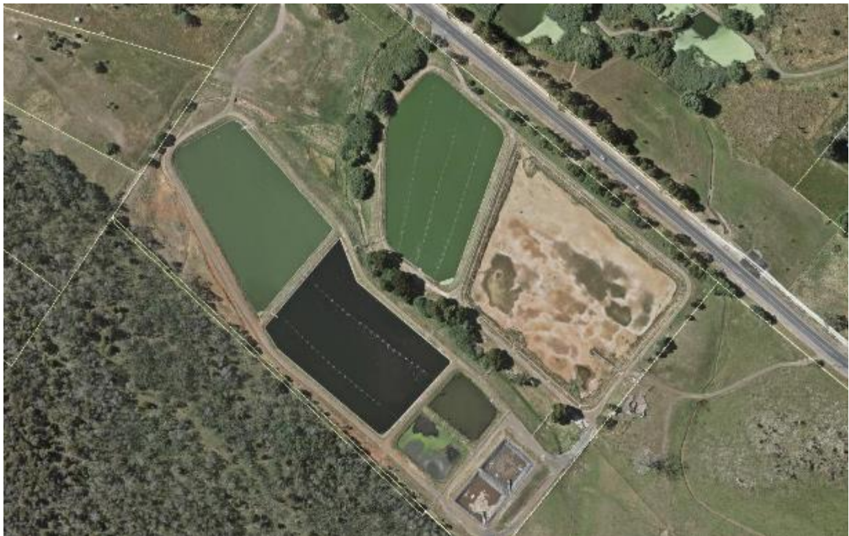
Figure 44-1: Prospect Vale Sewage Treatment Plant
