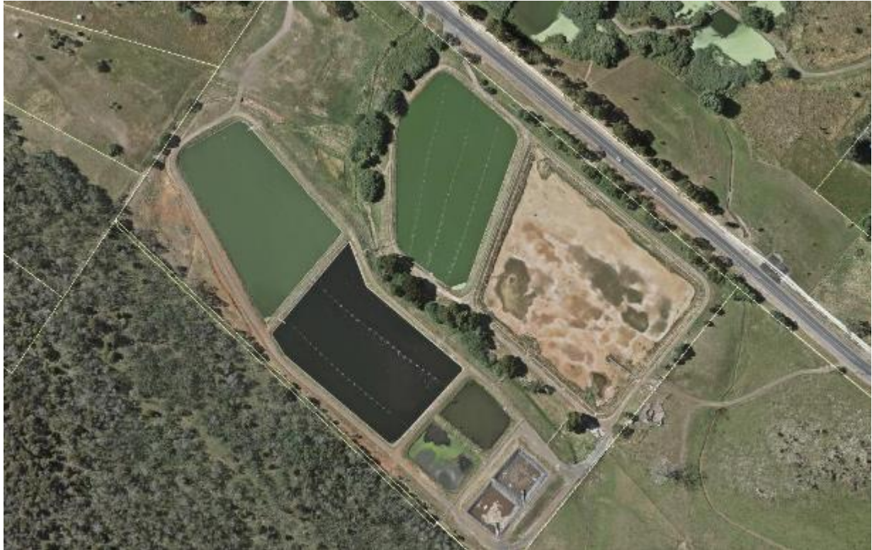
Figure 44-1: Prospect Vale Sewage Treatment Plant
