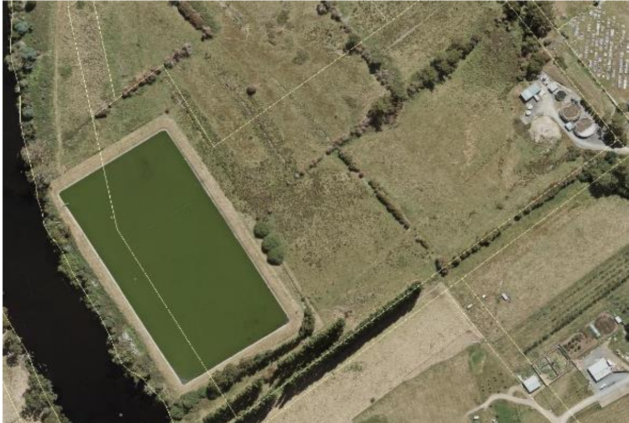
Figure 47-1: Ranelagh Sewage Treatment Plant
