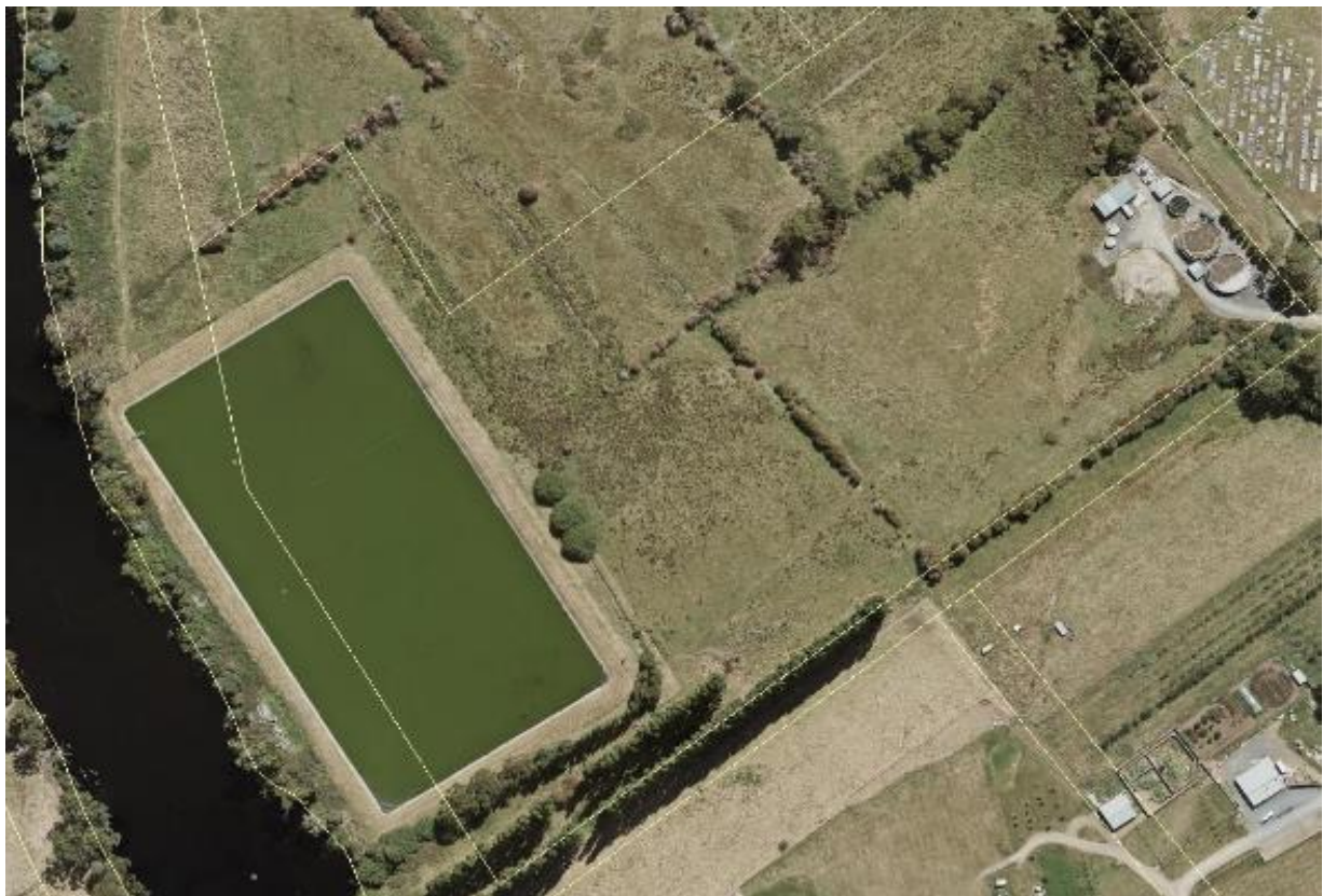
Figure 47-1: Ranelagh Sewage Treatment Plant
