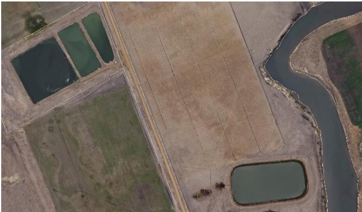
Figure 48-1: Richmond Sewage Treatment Plant
