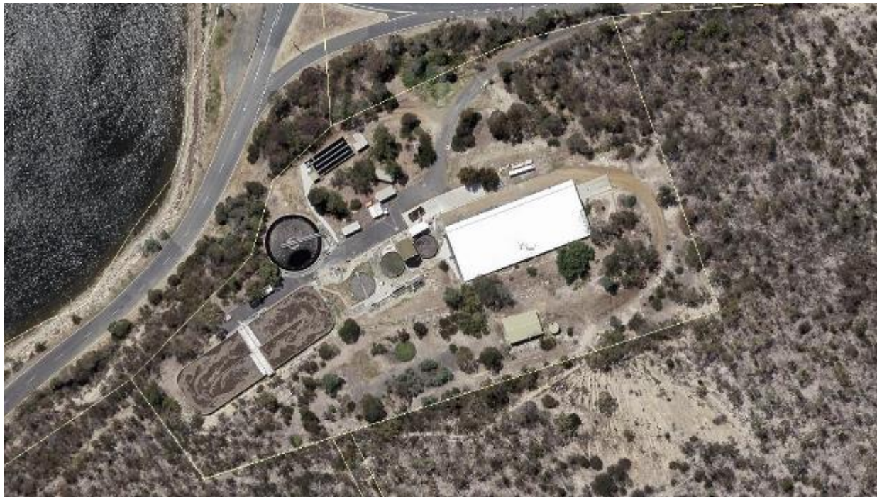
Figure 50-1: Risdon Sewage Treatment Plant
