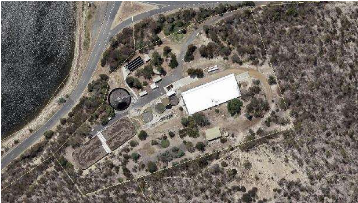
Figure 50-1: Risdon Sewage Treatment Plant
