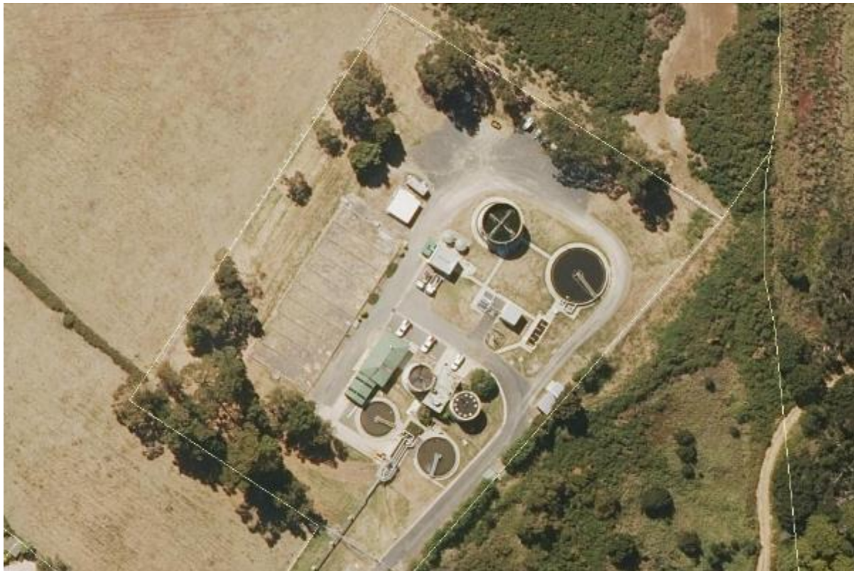
Figure 51-1: Riverside Sewage Treatment Plant
