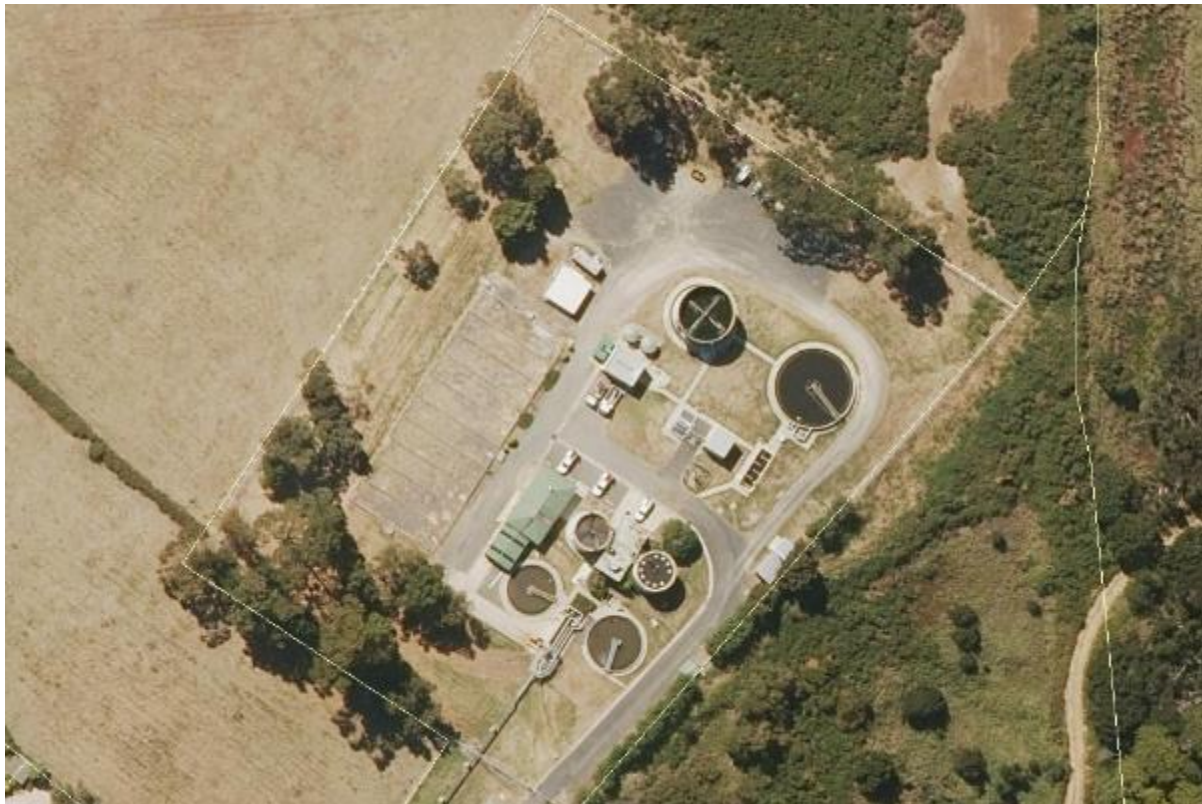
Figure 51-1: Riverside Sewage Treatment Plant
