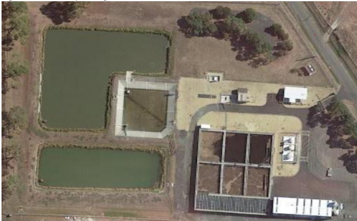
Figure 52-1: Rokeby Sewage Treatment Plant
