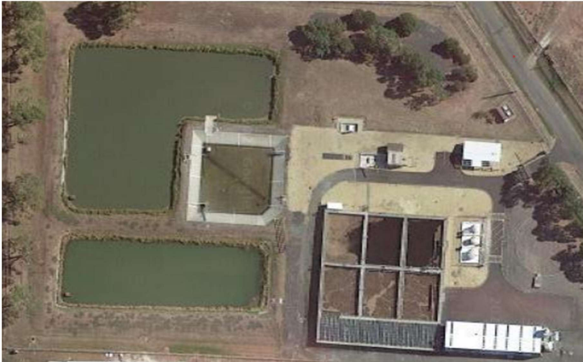
Figure 52-1: Rokeby Sewage Treatment Plant
