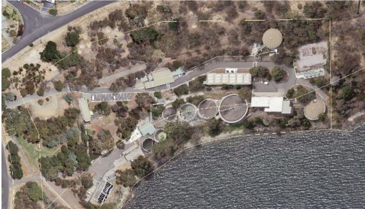
Figure 54-1: Rosny Sewage Treatment Plant
