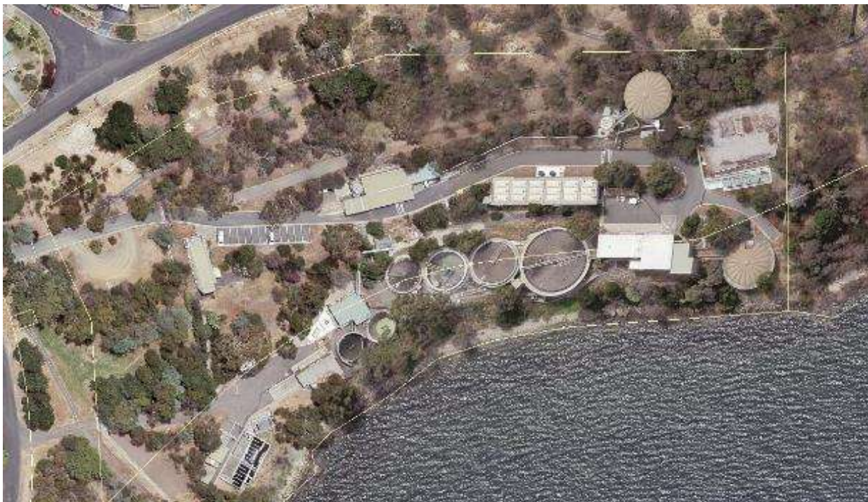
Figure 54--1: Rosny Sewage Treatment Plant
