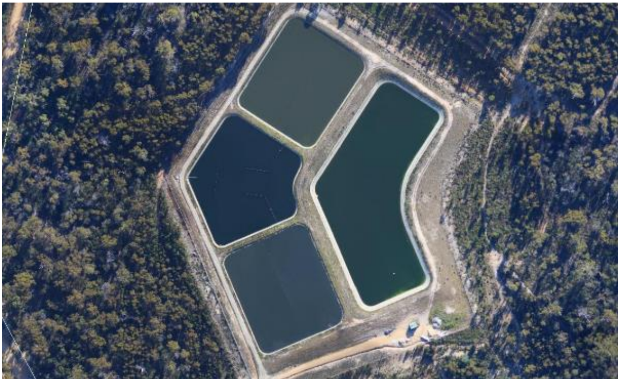
Figure 55 -1: Scamander Sewage Treatment Plant
