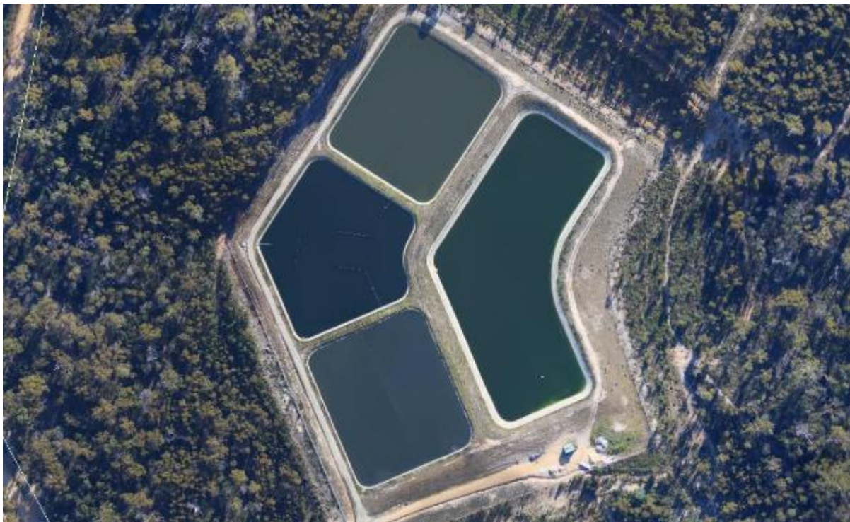
Figure 55 -1: Scamander Sewage Treatment Plant
