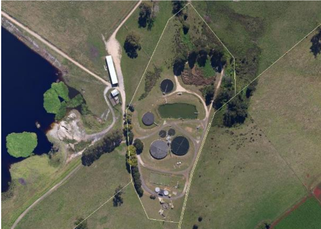
Figure 56-1: Scottsdale Sewage Treatment Plant
