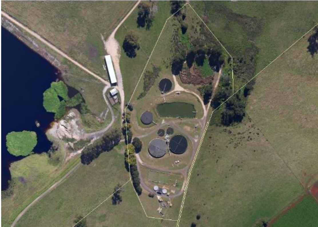
Figure 56-1: Scottsdale Sewage Treatment Plant
