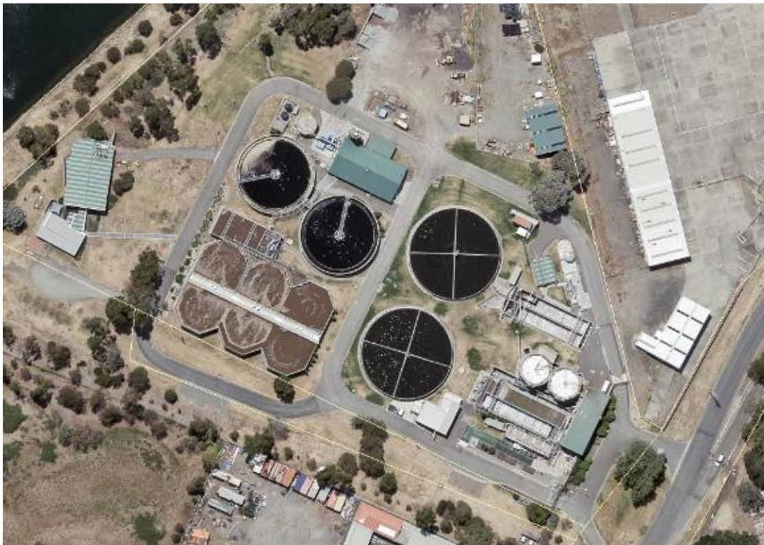
Figure 57-1: Selfs Point Sewage Treatment Plant
