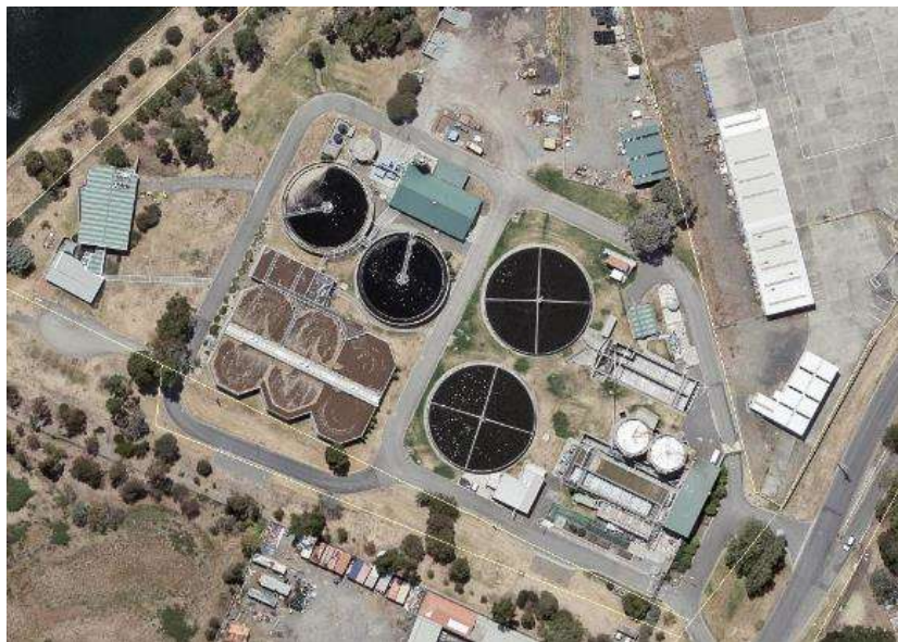
Figure 57-1: Selfs Point Sewage Treatment Plant
