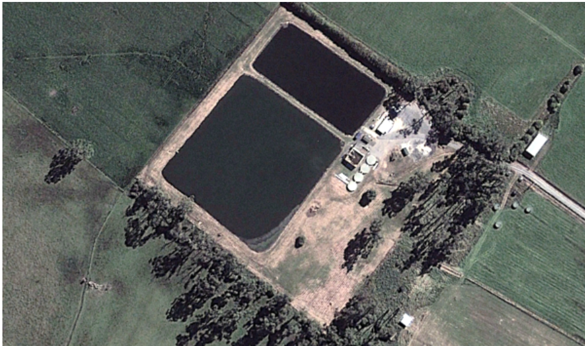
Figure 58-1: Sheffield Sewage Treatment Plant
