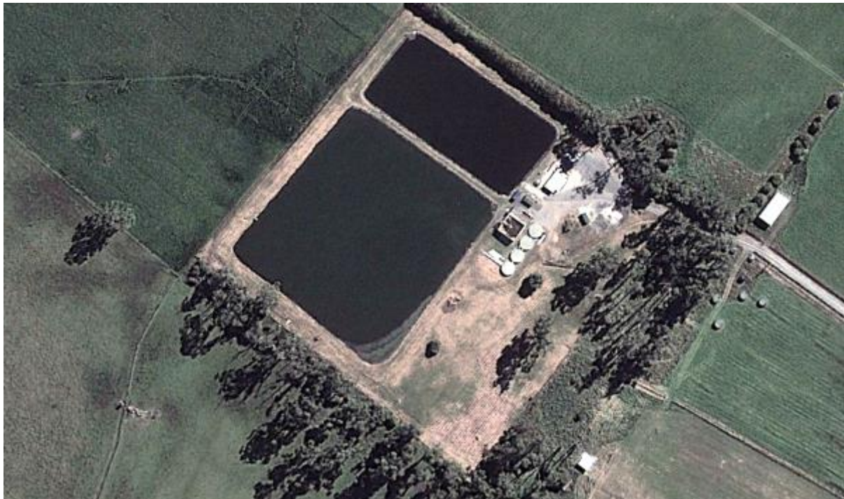
Figure 58-1: Sheffield Sewage Treatment Plant
