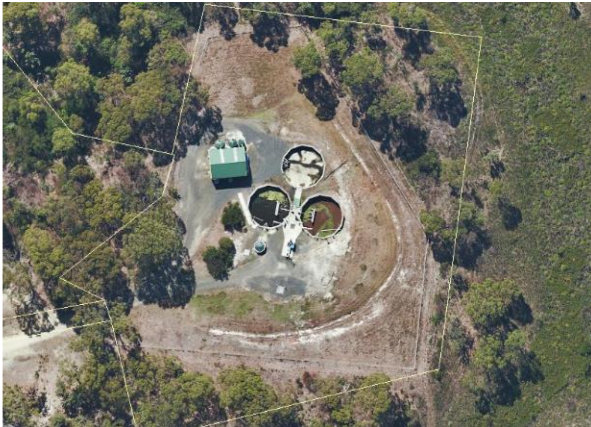
Figure 59–1: Sisters Beach Sewage Treatment Plant
