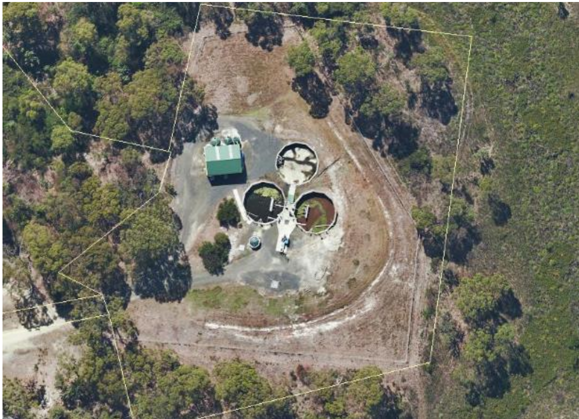
Figure 59–1: Sisters Beach Sewage Treatment Plant
