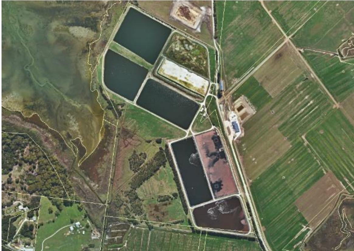
Figure 60-1: Smithton Sewage Treatment Plant
