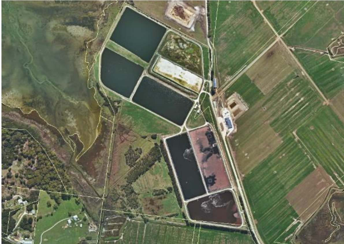
Figure 60-1: Smithton Sewage Treatment Plant
