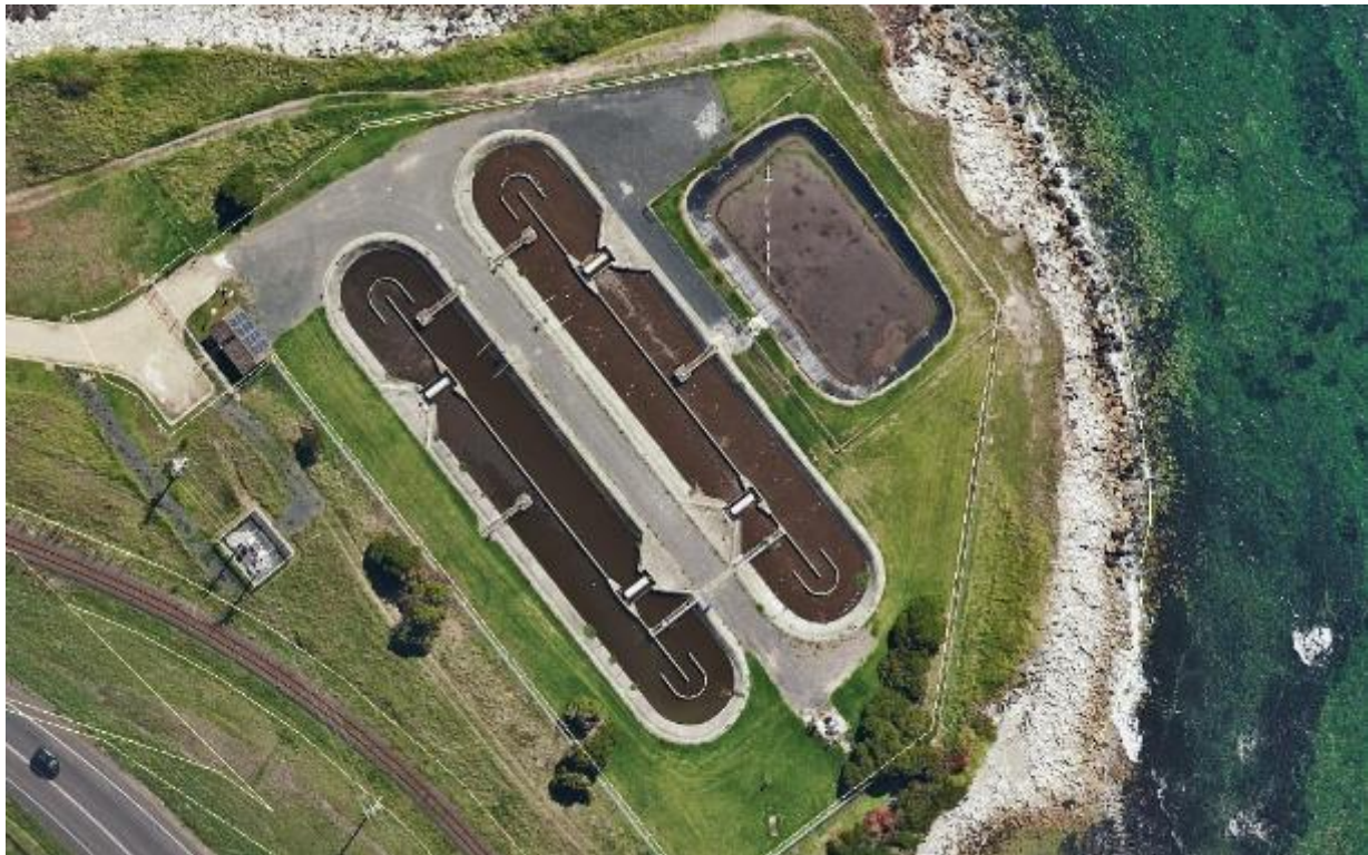
Figure 61-1: Somerset Sewage Treatment Plant
