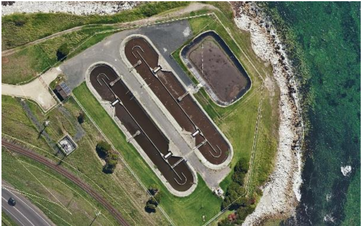
Figure 61-1: Somerset Sewage Treatment Plant
